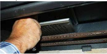
Loosen bolts on catalyst retainer, slide the catalyst retainer to the right to remove.
