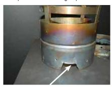
Install flex liner into existing chimney as per liner manufacturer's specifications. Ensure that the notch on the adapter cut in the previous step is pointed forward at about the 6 o'clock position. See Diagram 1.
