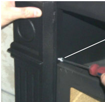
Secure top of faceplate with screw.
