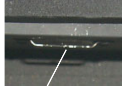
Bracket inside top of firebox.
