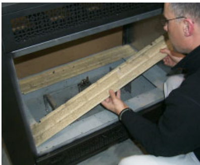
Remove the 2 Long Base Brick Panels
