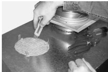
Remove the 2 screws holding the cover plate on the fireplace side.
