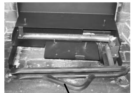
Front Burner Removed
