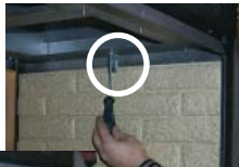
Remove the 2 Long Base Brick Panels
