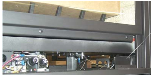
Remove cover to access Terminal Block
