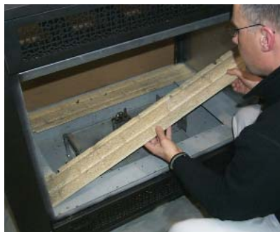
Remove the 2 Long Base Brick Panels
