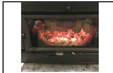
Typical Low Fire Coal Bed
