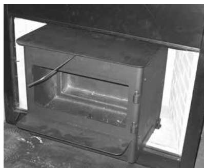
Diagram 5 Pull Rod In Place
